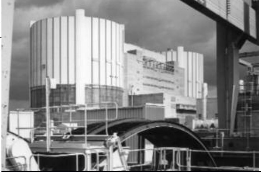
The ageing Magnox power station at Oldbury: due to be decommissioned this December.
