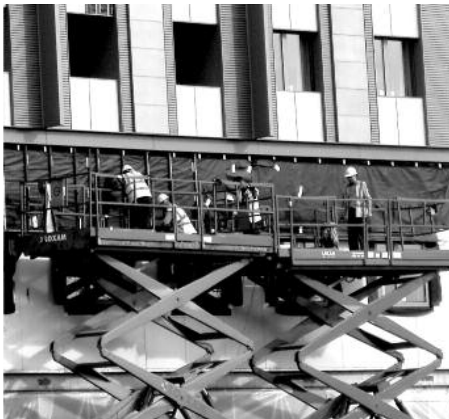
High-rise student accommodation under construction at Tottenham Hale, North London
