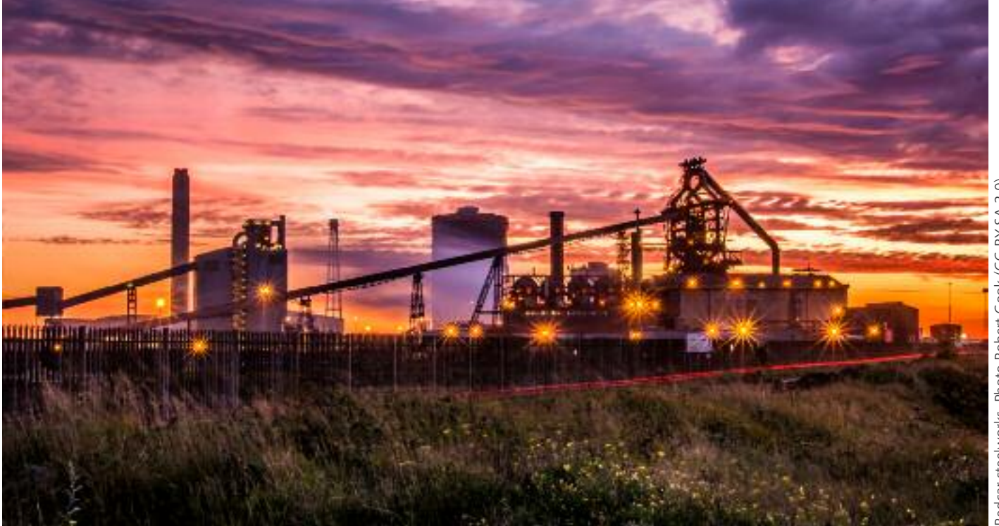
Redcar steelworks. Photo Robert Cook (CC-BY-SA 2.0)
