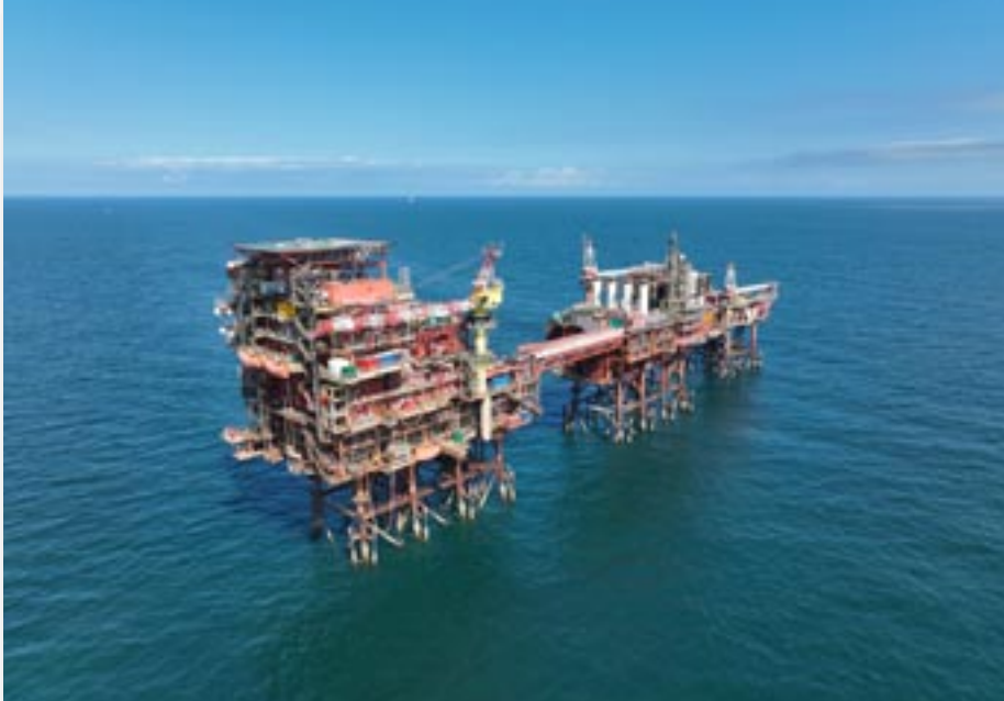
The Rough storage facility in the North Sea off Easington, Yorkshire.
