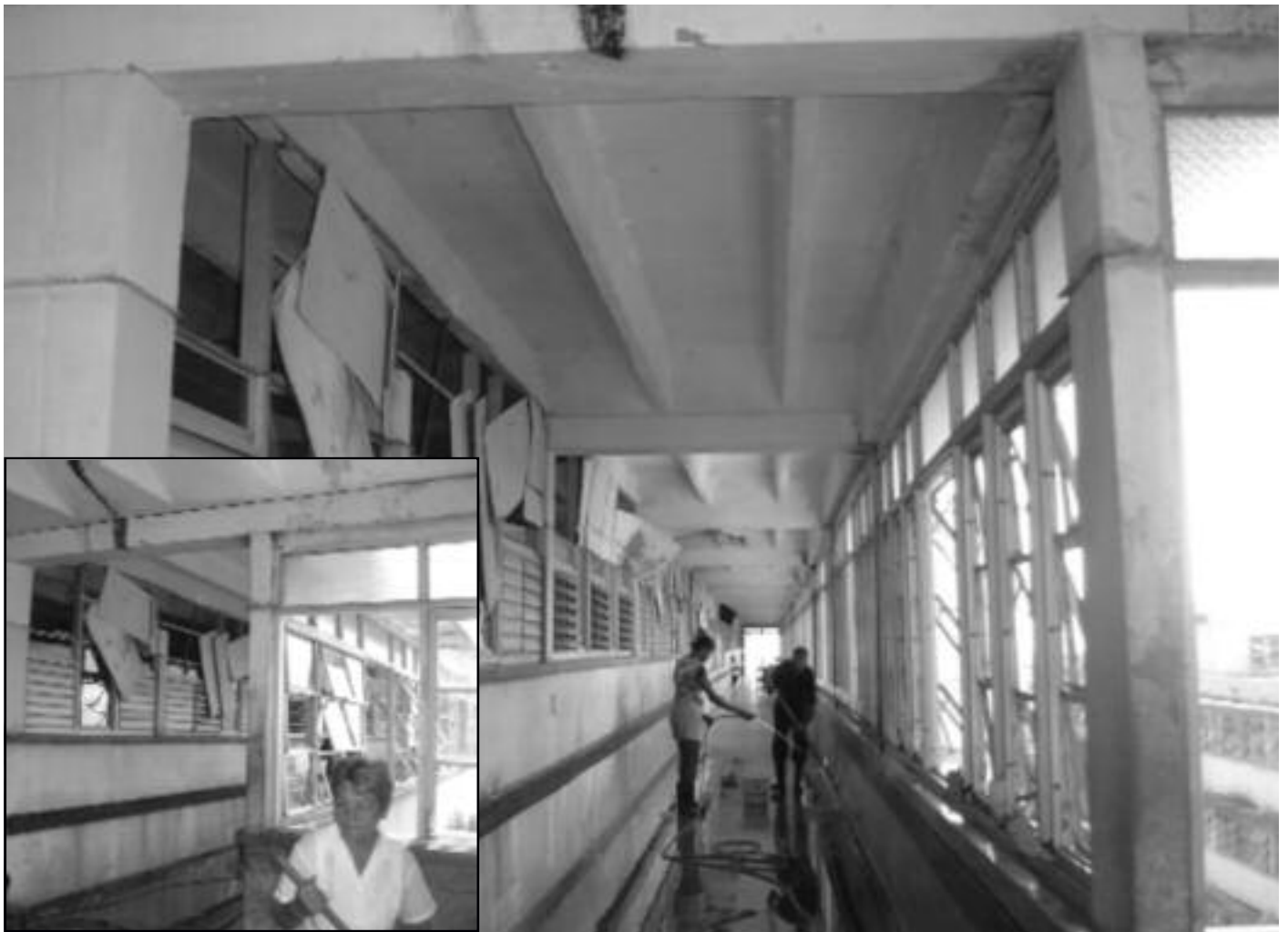
Clean up in the San Cristobal Hospital, Pinar del Rio, where 26 hospitals were badly damaged.
