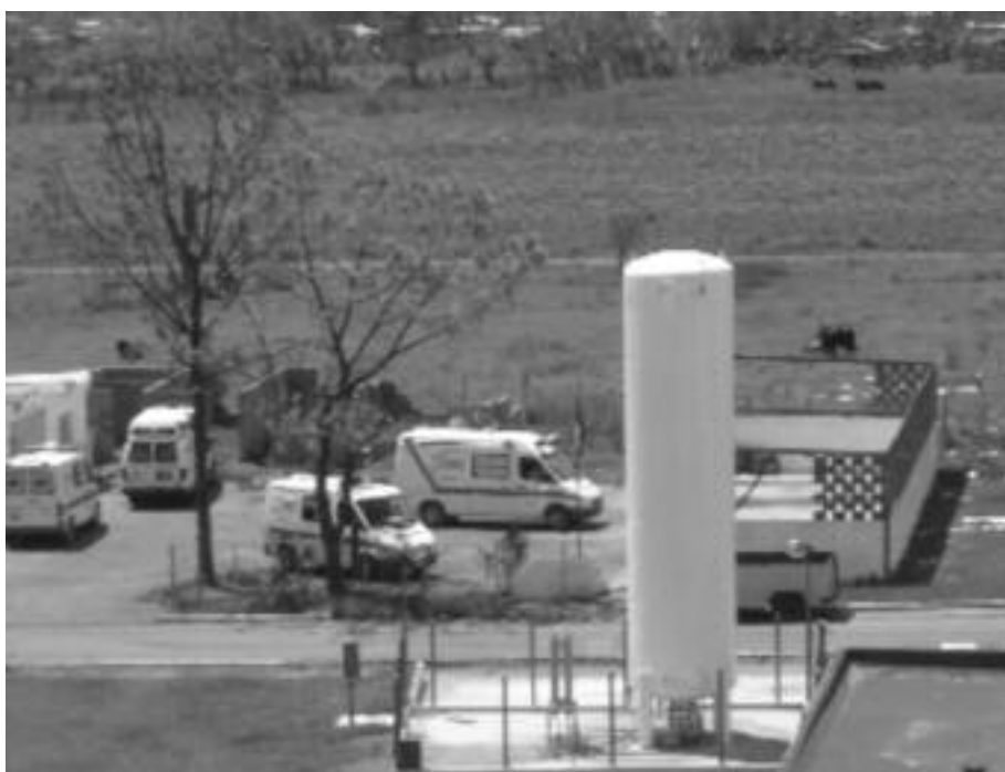
Ambulance station, Pinar del Rio – with the roof blown off.
