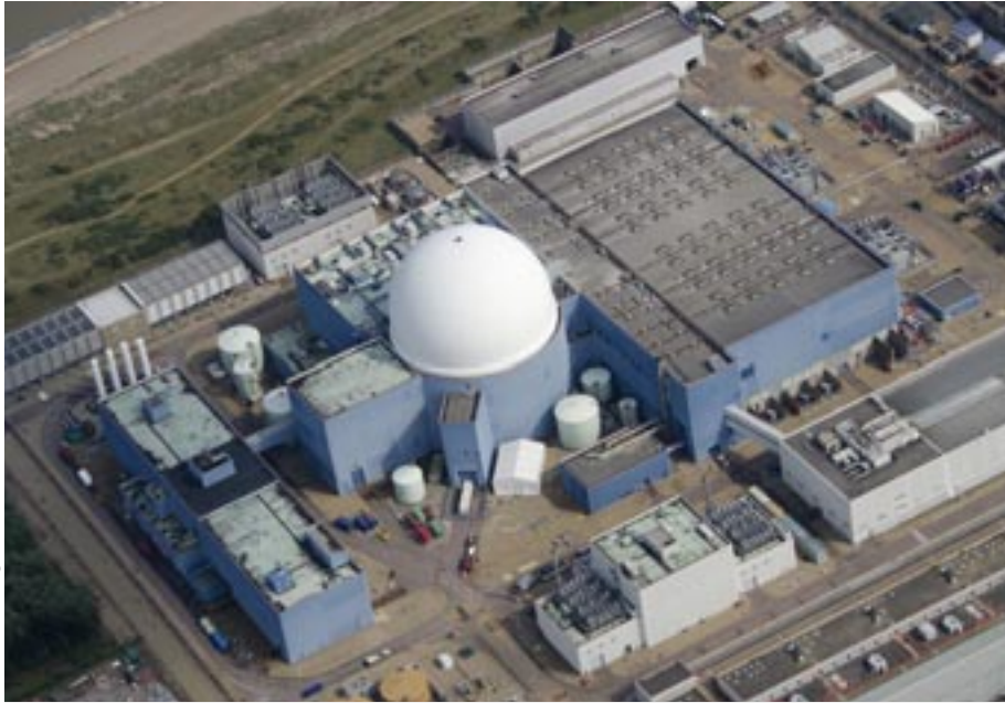
Sizewell B nuclear power station, Suffolk.
