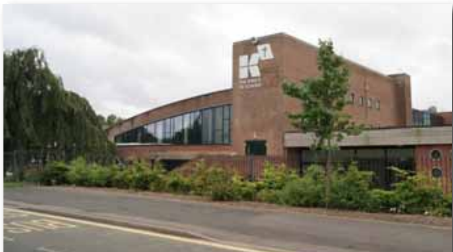
King's Church of England Secondary School in Tettenhall, Wolverhampton.
